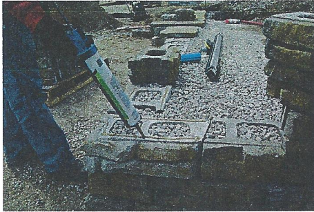
13. Clean block and apply optional adhesive for Copings. If Freestanding courses are to be placed on top of wall, connect to Retaining blocks per design details.
