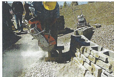
11. Trim blocks as required and remove knobs on top course to prepare for coping or Freestanding Block.
